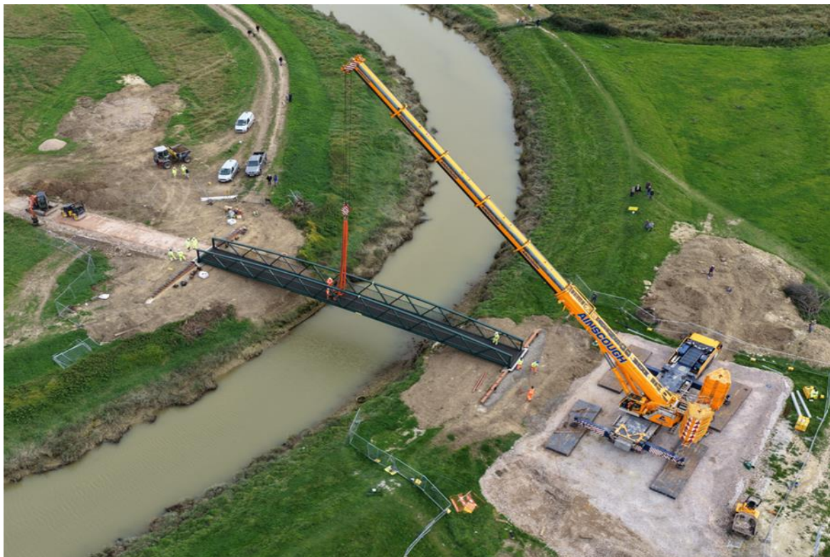
Aerial photograph showing the new bridge being placed
