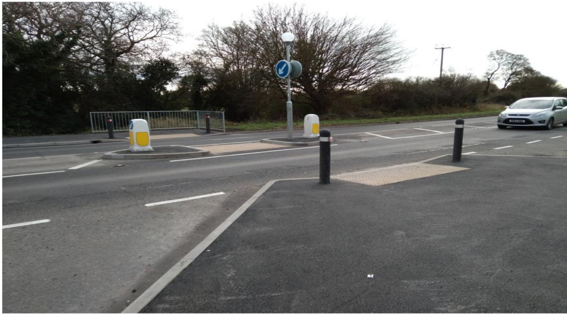
Image of improvements to the dropped crossing, splitter island and additional pedestrian guard rail outside Hunston Community Club
