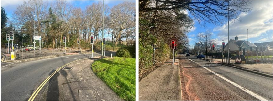
Refurbished Traffic Signal and crossings at Haslett Avenue East / Hawth Avenue, Crawley
