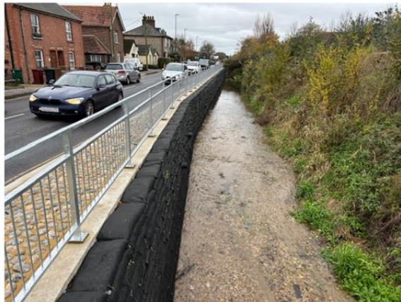
Image 1. Environmentally friendly "FlexMSE" soil bagwork
