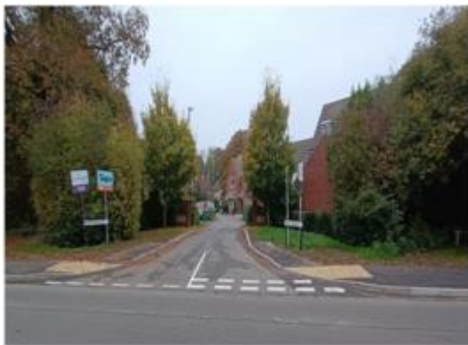
A new uncontrolled pedestrian crossing at the entrance to Martindales and the installation of road markings at this junction.
