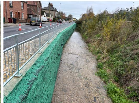
Image 2. Hydroseeds in green colour to make application visible. The seeds are coated with water gel before spraying onto the bagworks.
