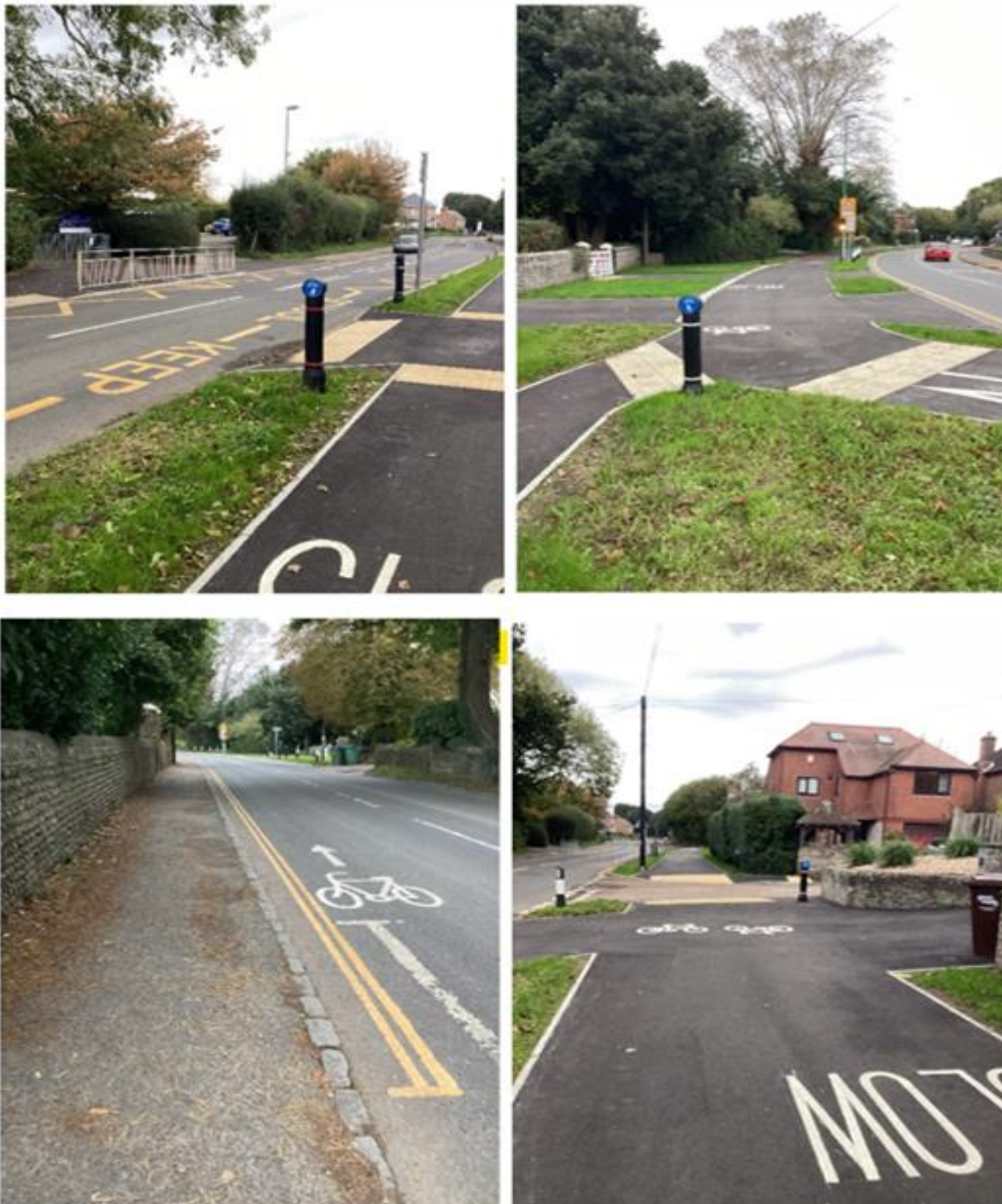
A new shared pedestrian and cyclist path near Yapton Primary School
