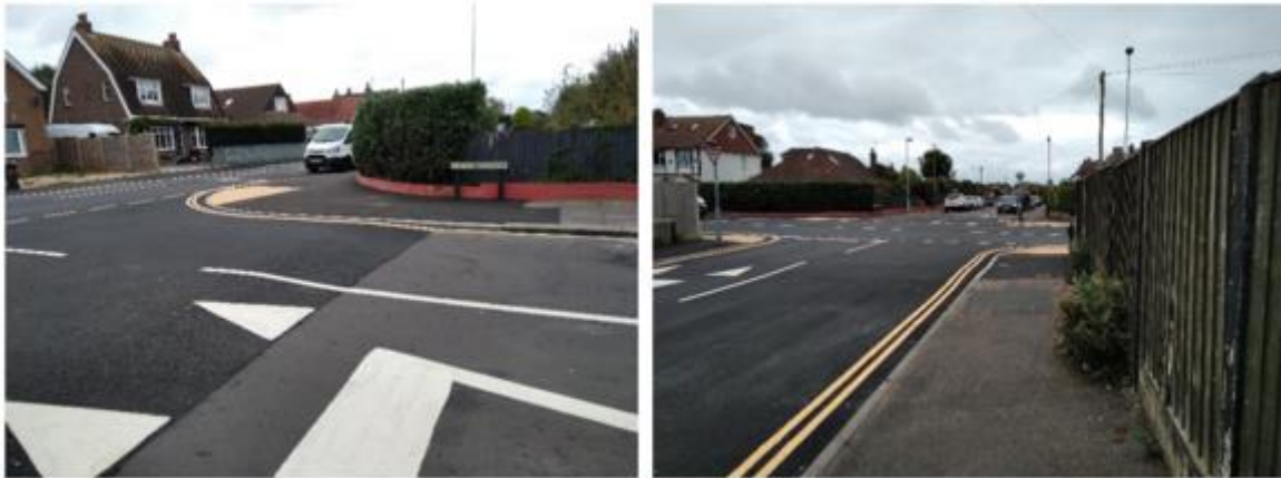
Tactile crossing points and double yellow lines at junctions and refresh lining at Cotswold Road and Salvington Road, Worthing
