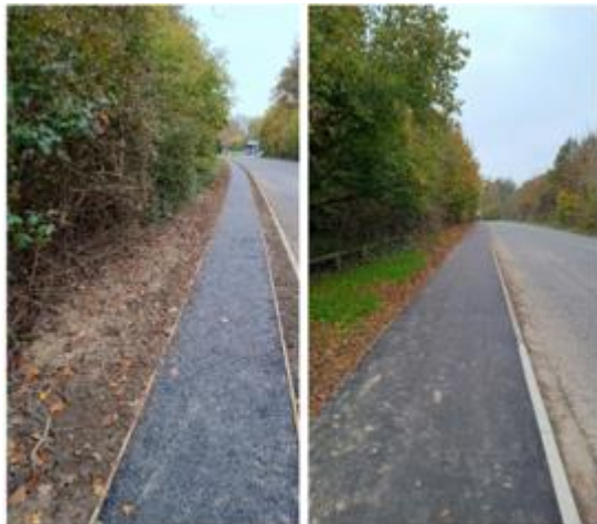
Above Image: New pedestrian footpath within the Western verge of the Blakes Farm Road between the southern roundabout with Wilberforce Way and the northern roundabout with Worthing Road.
