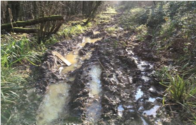
Restricted Byway 639 'Before'
